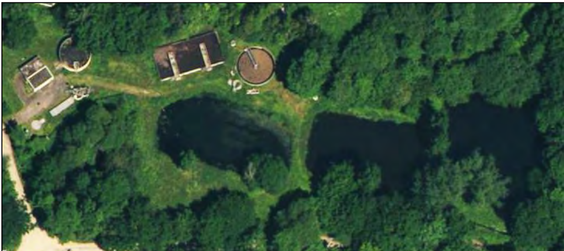
Figure 26 : Station d'épuration de Brouelic, Ile aux Moines
